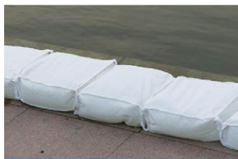
Place First Row of Bags Down, With the Long Side Parallel to Water
