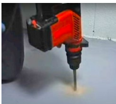
Drilling For Mounting
